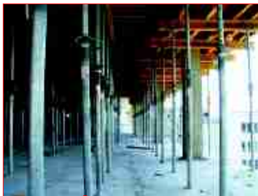
H-beams on the cross head
