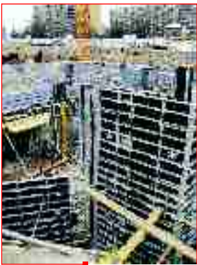
Building site — MIDI BOX
