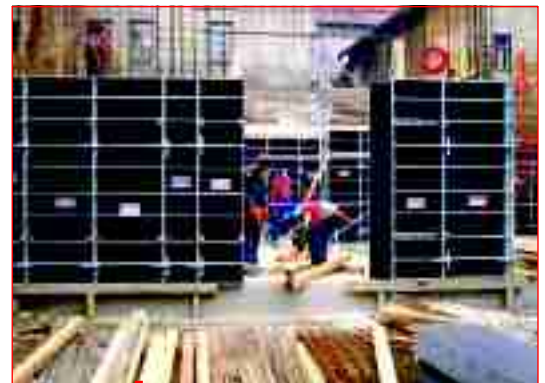
MIDI BOX formwork — building site in Sarajevo
