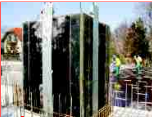
Formwork removal of the lift shaft formwork
