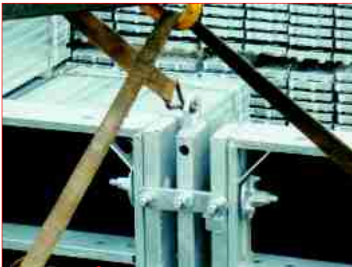
Formwork removal of the lift shaft formwork
