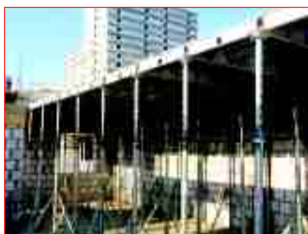
ALUstrop on building site
