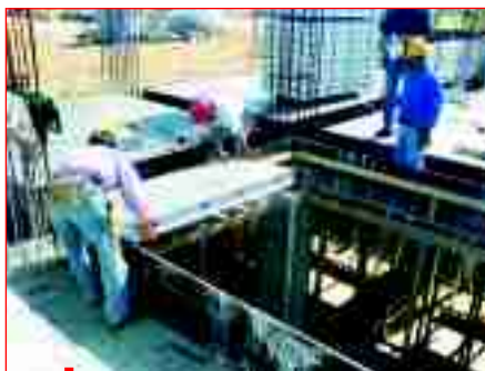
ALUstrop board during assembly
