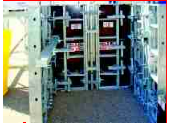
Lift shaft formwork
