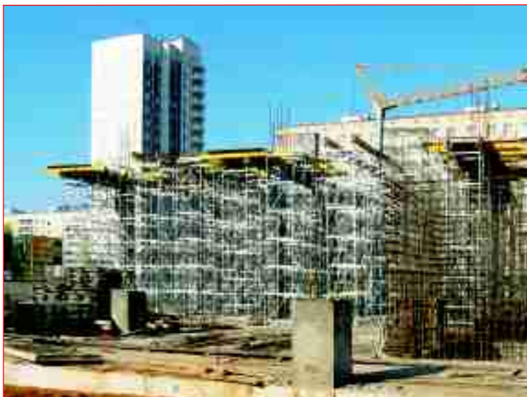
S10 tower – realization of a monolithic building structure formwork
