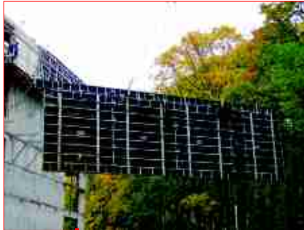
MIDI BOX PLUS shuttering boards – building site
