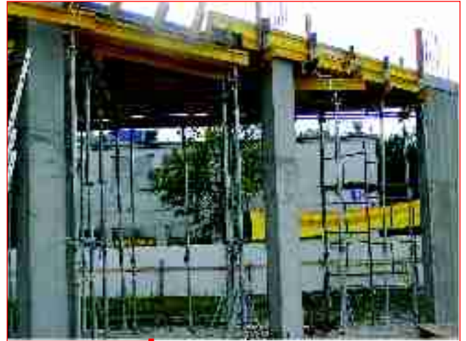
Support and tripod application on the building site
