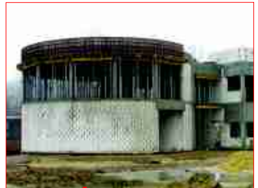
Ceiling formwork application on the building site
