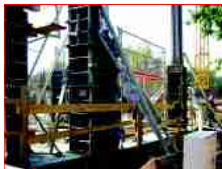
Pole forming – MIDI BOX boards and BM260 locks
